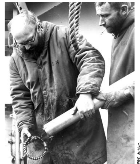
British oceanographer John Swallow, left, and Gordon Volkmann of WHOI prepare a pinger for a Swallow float aboard Erika Dan in 1962. Swallow received WHOI's Bigelow Medal that year. The citation said the Swallow float "has become the principal tool for the study of deep water circulations. The results of these studies have revolutionized our conceptions of the character of the deep water motions. Instead of the sluggish, widespread drift anticipated from continuity considerations, the deep layers seem to be moving briskly and not in accordance with any known process. Here then, is a scientific fact that challenges the imagination."
